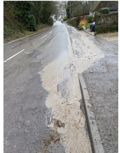
Blocked gully at 27 Oxford St
